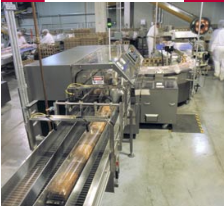
▲ To keep up with oven speeds, Pepperidge Farm turned to flow-wrapping for its signature inner wrap on sliced bread. Loaves then feed into a dual-lane bagger.
